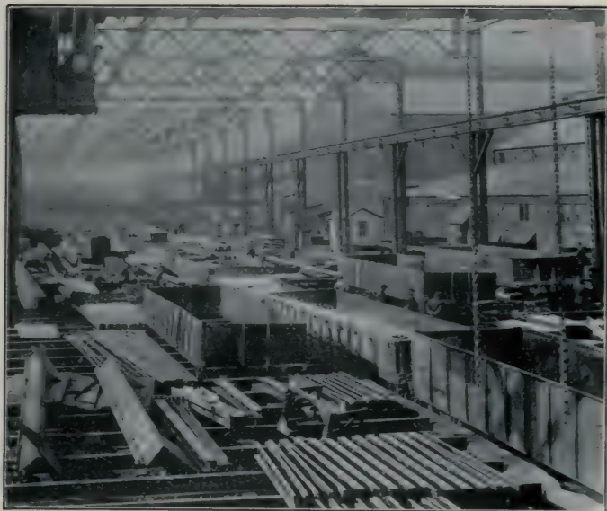
STRUCTURAL MILL, LOADING YARD AND STOCK YARD, HOMESTEAD WORKS, CARNEGIE STEEL COMPANY
